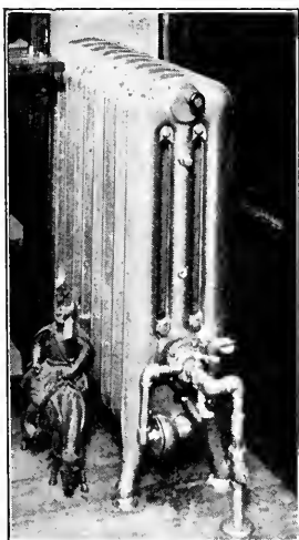
FIG. 1. TYPICAL UNVENTED GAS-STEAM RADIATOR
